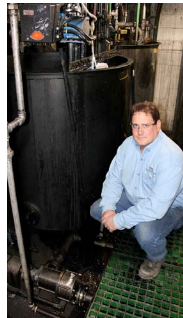
Tim Kreitz, Project Engineer at Rock-Tenn's St. Paul Paper Mill, kneels next to the Blackmer C-Series Eccentric Disc Pump.
